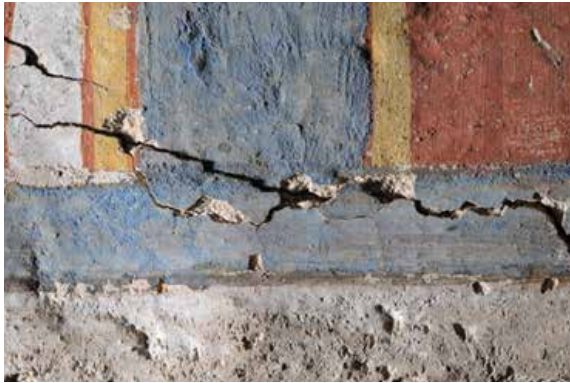
図9 彩色層に起きた剥離と亀裂 Fig.9 Flakings and cracks in the paint layer
